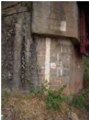
Water Gauge at Bridge Abutment, Route 9, Savannakhet Province
