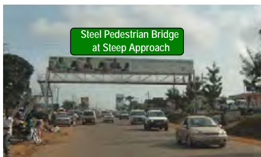
Exiting Pedestrian Bridge at Nakawa on Jinja Road Source: JICA Study Team
