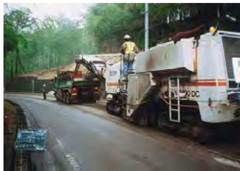
Cutting machine of the crawler type.
