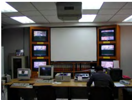
Traffic Control Center
