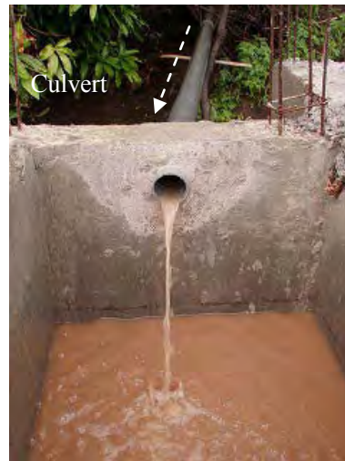
Left: Conditions of the catchment on the surface roads
