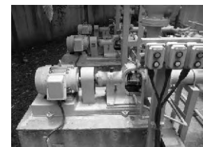
Figure 3.4.8 Return sludge pump
