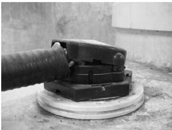
Figure 3.2.50 Water supply tank level switch terminal box
