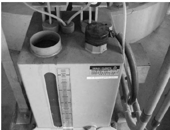
Figure 3.2.48 Chemical tank
