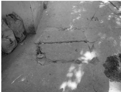
Figure 3.3.6 Man-hole with bad condition
