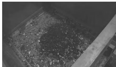
Figure 3.2.38 Removed grit
