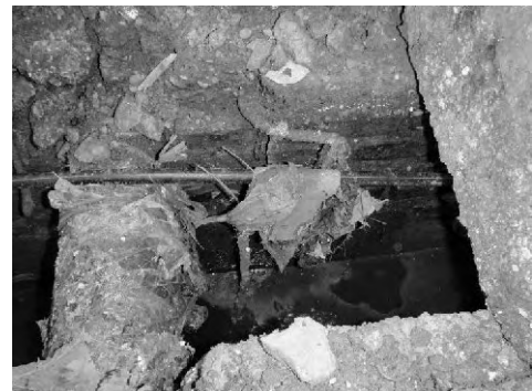
Figure 3.3.9 Ditch covered with sludge
