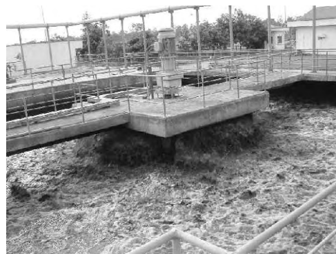
Figure 3.2.39 Under operation of aerator
