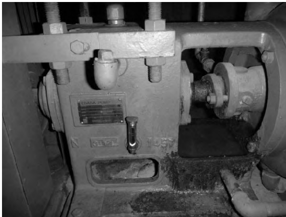
Figure 3.2.44 PST sludge pump
