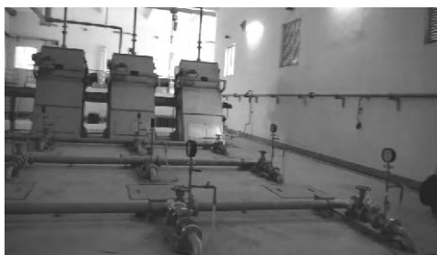
Figure 3.2.37 Grit removal facility
