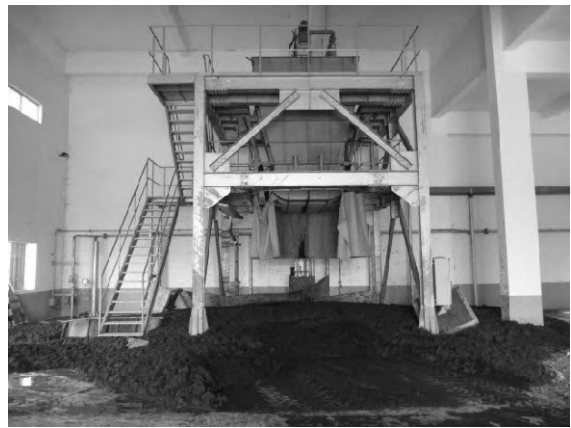
Figure 3.2.45 Sludge cake hopper
