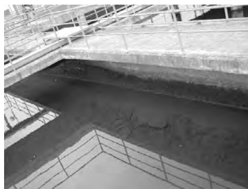
Figure 3.2.40 Surface at aerator stop timing
