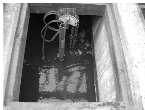
Figure 3.2.25 Equalization tank
