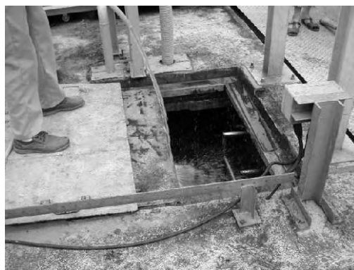
Figure 3.2.4 View of cleaning grit chamber
