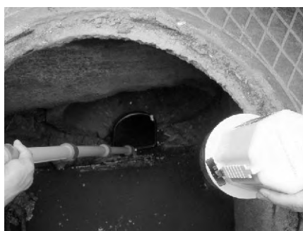
Figure 3.3.2 Sewer survey with mirror
