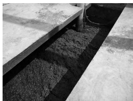
Figure 3.2.11 Filtrate return pit
