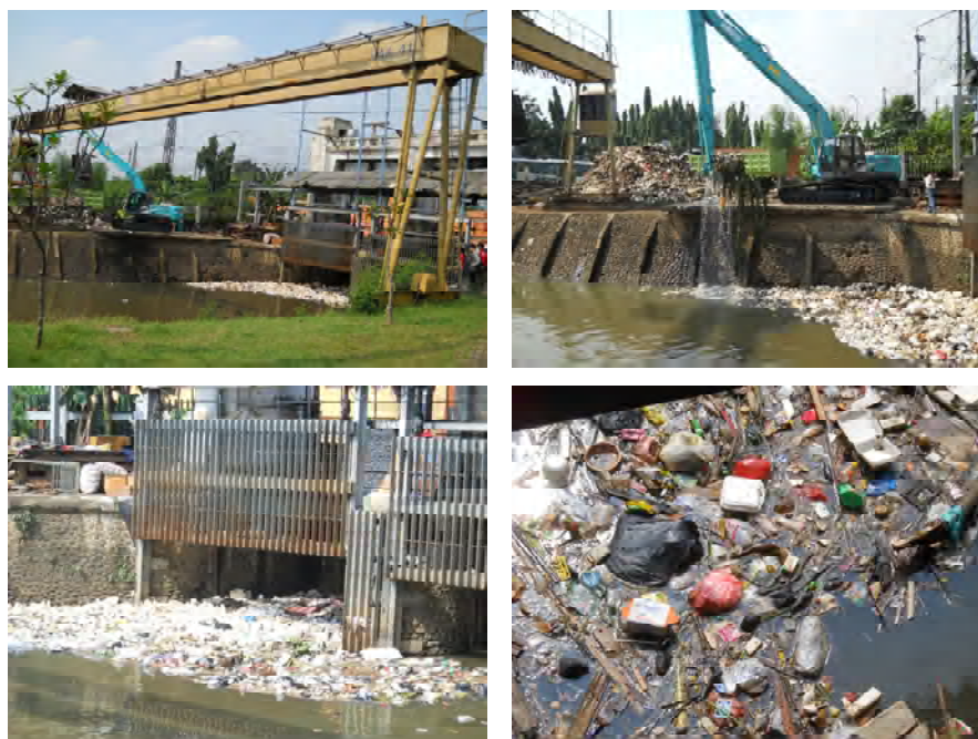
Fig. 4.5.4 Manggarrai Watergate (30 April 2010)
