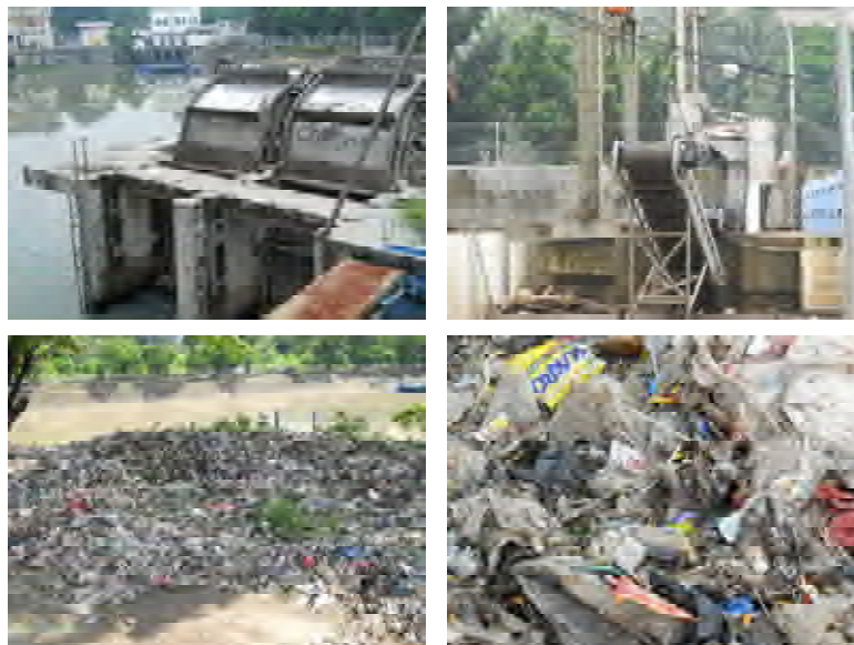
Fig. 5.1.1 Setiabudi waste treatment pond (May 2010)
