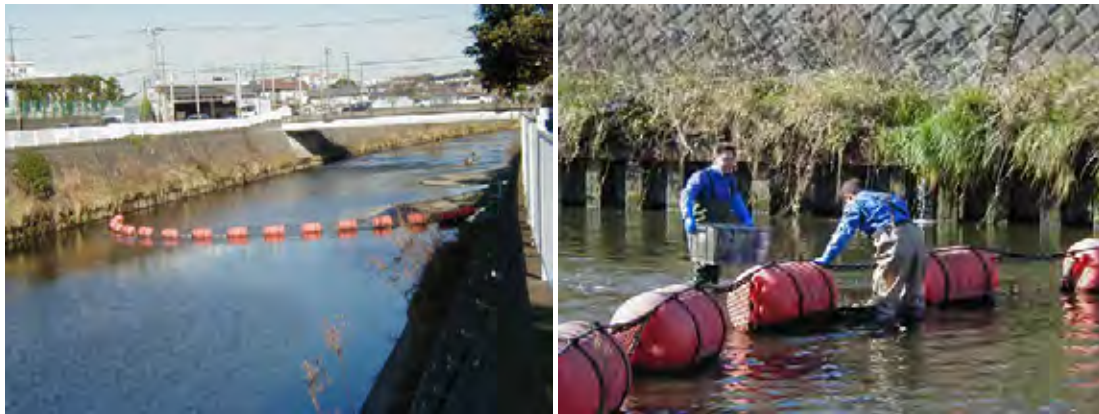
Fig. 5.1.5 Floats used as floating waste removal for Hikiji River, Fujisawa in Japan
