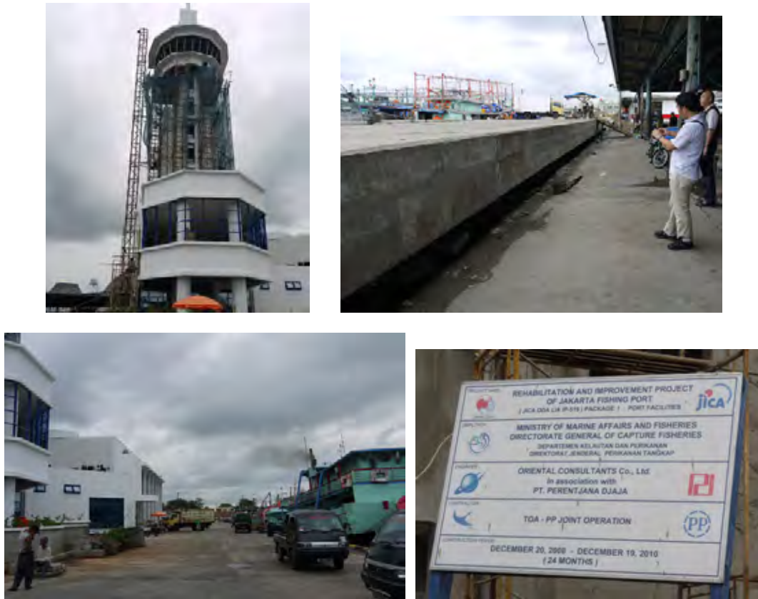
Fig. 4.2.13 Jakarta Fishing Port Improvement Project
