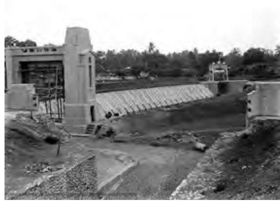
(b) West Canal constructed in 1920
