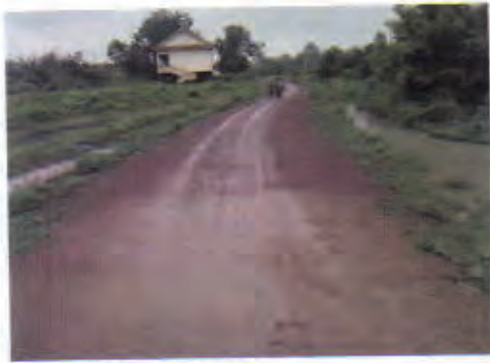
Constructed Road: No problem.
