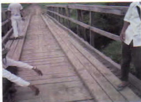
An example of the bridge construction project financed by Commune Fund: Material quality & size have a little difference from the pilot project.
