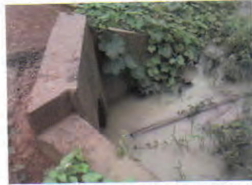
A culvert along the constructed road Installed by the commune
