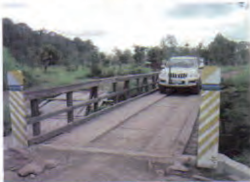
A new bridge: w3.5m/115m with the local standard, max. weight; 10t, 15 year duration, next to the old broken one
