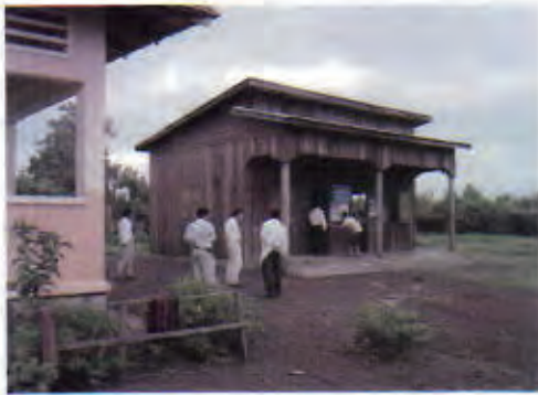
A new facility constructed by local standard (wooden structure with concrete floor & foundation) for the staff on night duty next to the District Health Post.
