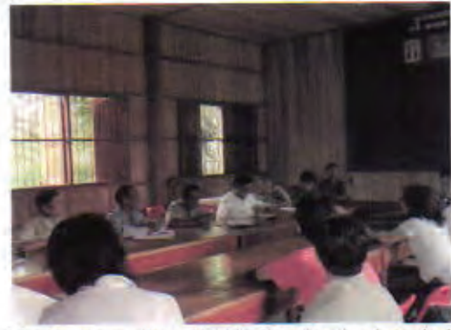
Meeting room with no finishing based on local standard. Wood materials had needed more time to dry if possible.
