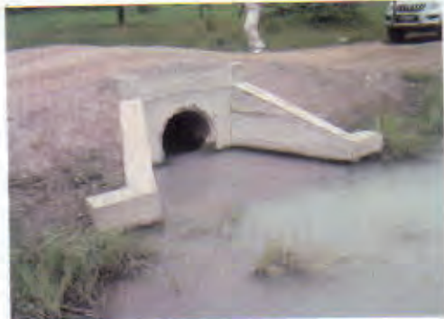
Culvert 5: No problem
