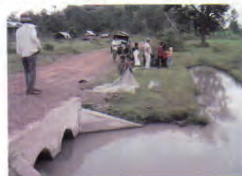
Culvert 3: No problem
