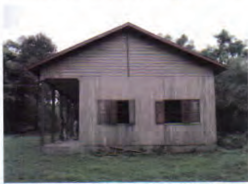
A new facility with library & meeting room for district. Wooden building with concrete floor & foundation.
