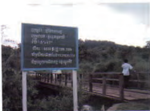
A signboard describing the pilot project at the side of the rehabilitated wooden bridge
