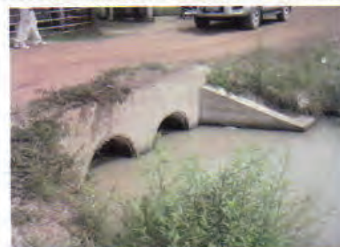
Culvert 1: No problem
