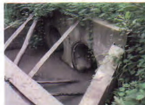
Culvert 4: No problem with its structure.
