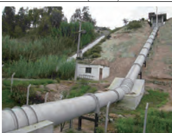
Mini-hydro project (Peru)
