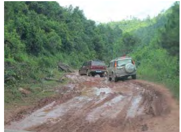
Road condition along proposed raw water transmission line
