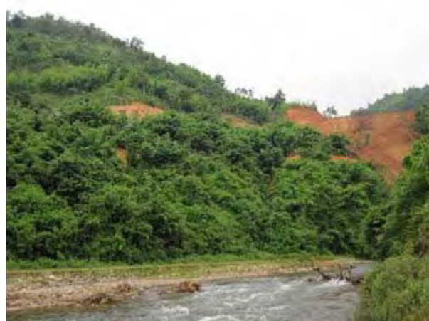
Location of proposed New WTP Q=1,000m 3 /day, located behind hill (subocular river is Nam Cau Spring)
