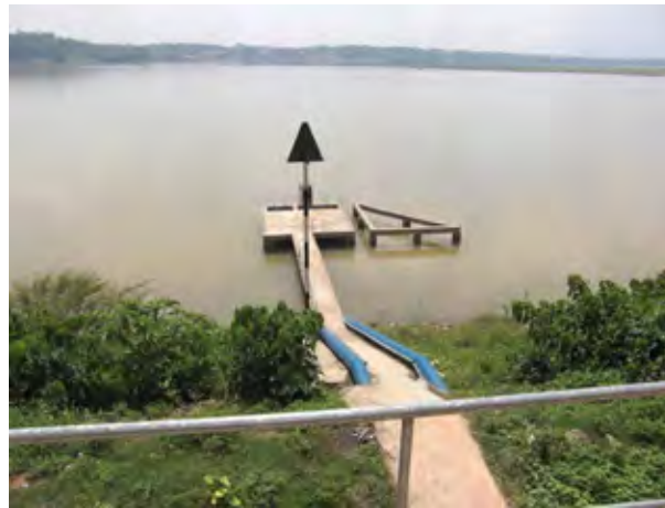
Existing intake facility located at Da river
