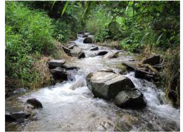
Location of proposed Intake Facility located at the right bank of Huoi Sang Spring, Q=600m 3 /day, by gravity (view from downstream)
