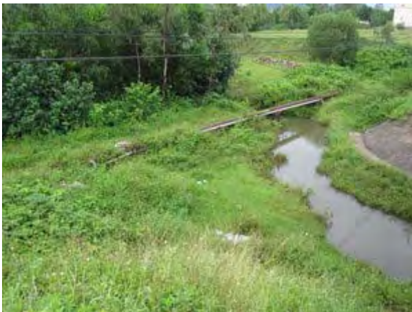
Location of proposed branch point of distribution main located the distance of around 5km from exist Vung Ang WTP
