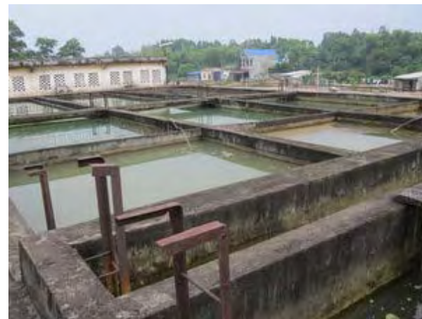
Exist. WTP would be upgraded under Norway fund from Q=15,000 to 20,000m 3 /day, which is water source of this Project
