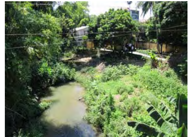
Exist. Intake Facility located at the right bank of Lu Stream, capacity would be upgraded (view from upstream)
