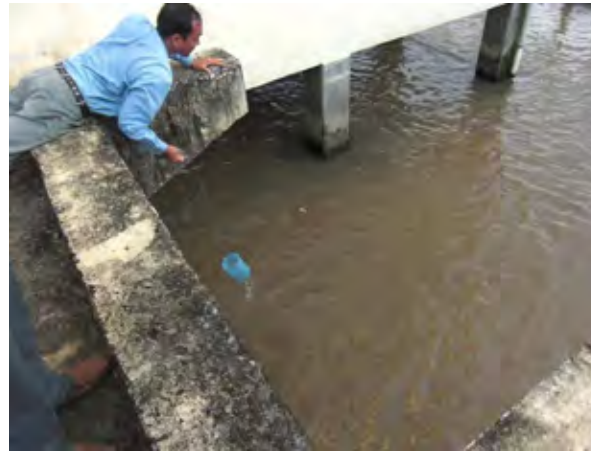
Water source Raw water in the water source is treated in existing water treatment plant and supplied to project area.
