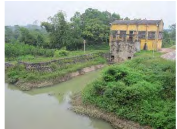
Exist. Intake Facility located at the left bank of Song Cong River, capacity would be upgraded under Norway fund (view from downstream)
