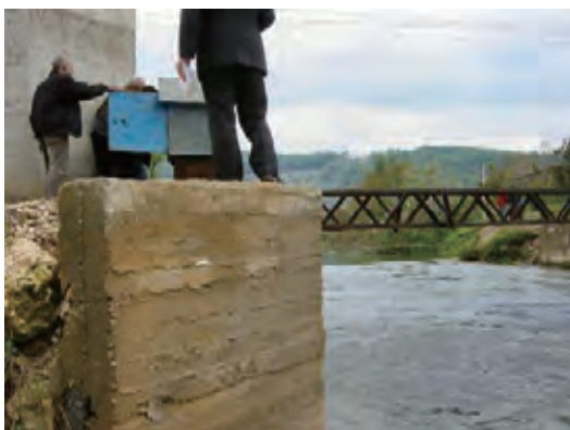
[WRIC018] "Al Sin" Automatic Water Level Station
