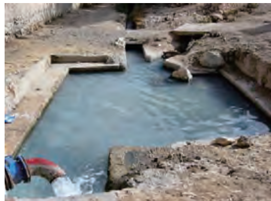
[WRIC009] Release Point of Pumped-up Water to Roman Irrigation Canal (Source of Water: "L9" Well)
