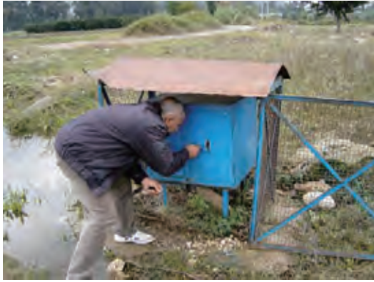
[WRIC020] "Al Sin" Automatic Observation Well - Water Level and Quality -
