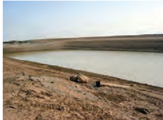
[WRIC032] "Saikel" Water Harvesting Reservoir Candidate surface water level observation site in WRIC Phase II.
