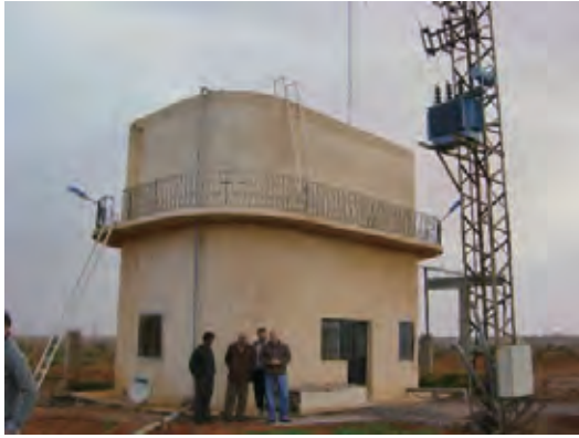
[WRIC003] "Al Sawra" Pumping and Distribution Station
