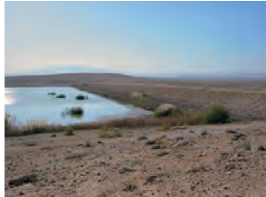
[WRIC024] Sadad Dam Storage Capacity: 2,000,000 m 3
