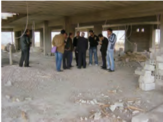
[WRIC005] WRD Data Center in Sweida (Under Construction)
