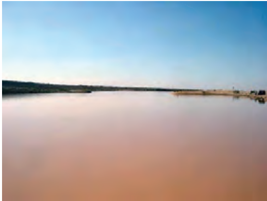
[WRIC023] Water Harvesting Reservoir (Name is not confirmed) Storage Capacity: 30,000 m 3
