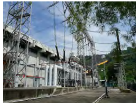
Gambar 3.6-12 Protection relay room Gambar 3.6-13 Trafo Utama 16.5/500kV
