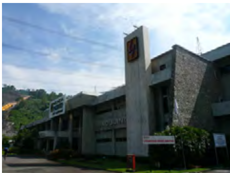
Gambar 3.6-8 Saguling hydropower plant
