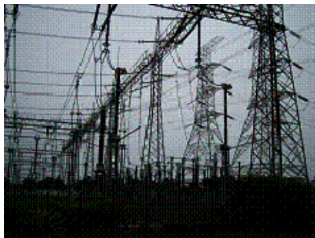
Figure 3.6-18 500kV transmission facility
