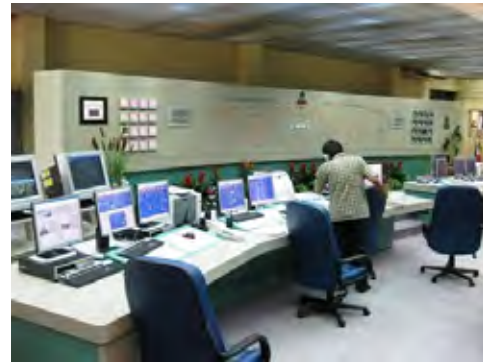
Figure 3.6-6 Central operation room
