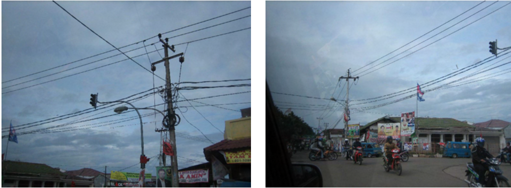
Figure 3.6-25 20kV distribution facility of the Jakarta suburbs
