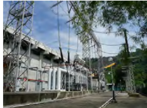
Figure 3.6-13 16.5/500kV main transformer
