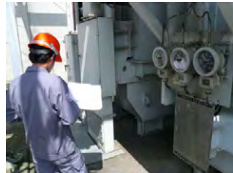
Figure 3.6-15 Situation of an inspection
