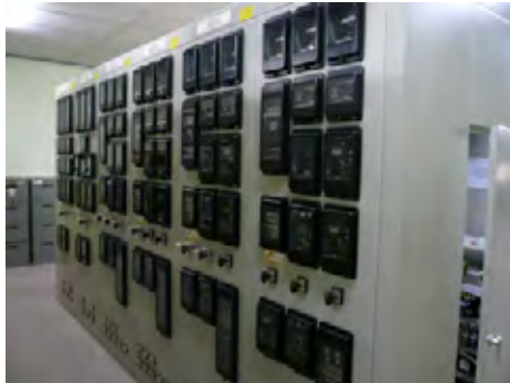
Figure 3.6-12 Protection relay panel
