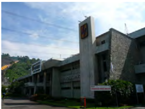
Figure 3.6-8 Saguling hydropower plant
