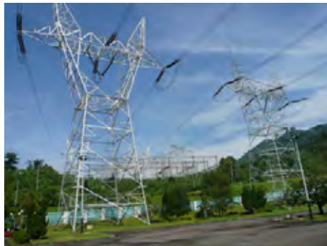
Figure 3.6-14 500kV Switching station
