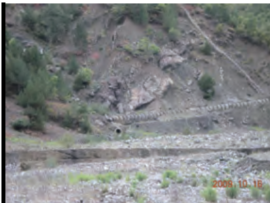
Photograph 5.6.13 Drain pipe (hillside) at No.3 tailings dam
