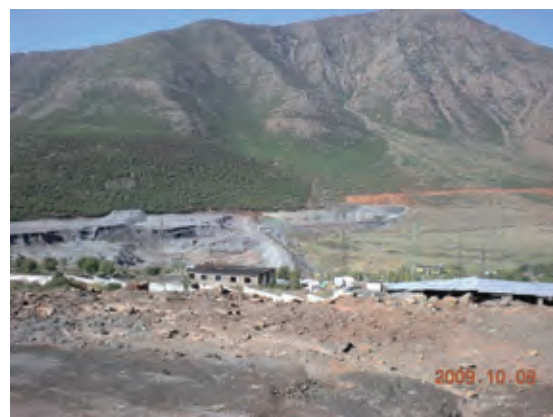
Photograph 5.6.2 Old tailings dam (left side) and new tailings dam (right side)
