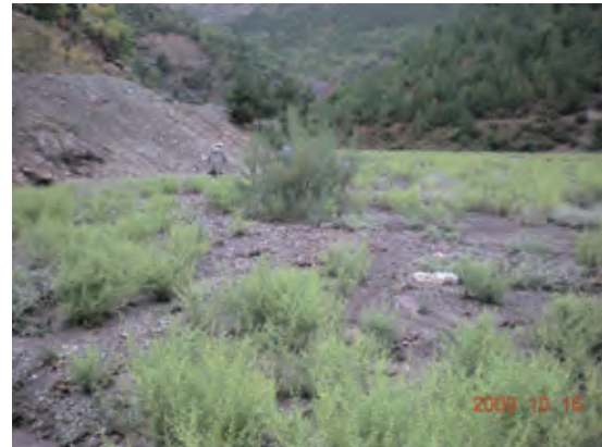
Photograph 5.6.12 Upper part of No.3 tailings dam and vegetation on the dam
