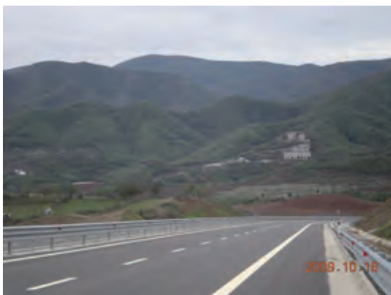
Photograph 5.6.15 Concentrator of Rreshen Cu mine
