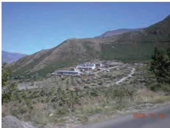
Photograph 5.6.1 View of Bulqiza concentrator
