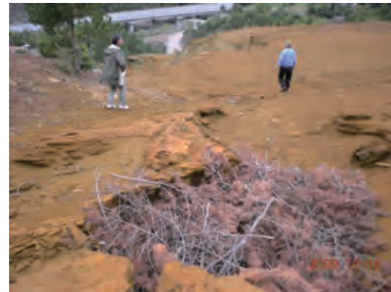
Photograph 5.6.14 Slope erosion at dyke of No.3 tailings dam
