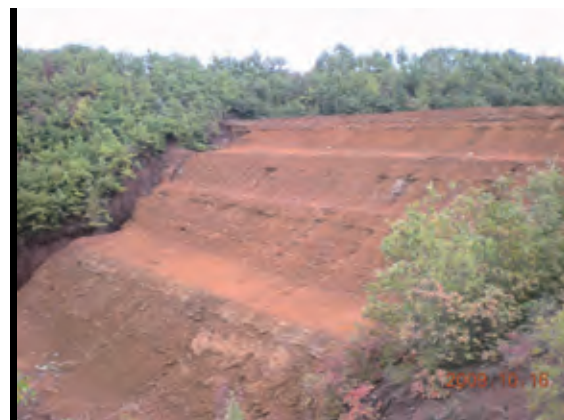
Photograph 5.6.16 Dyke of tailing dam
