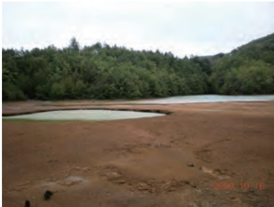
Photograph 5.6.17 Two caves occur in the tailings dam side of dyke (approximately 20 m in diameter, filled with water)
