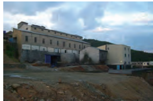
Existing copper ore concentration plant at Fushe Arrezi near Pukë.
