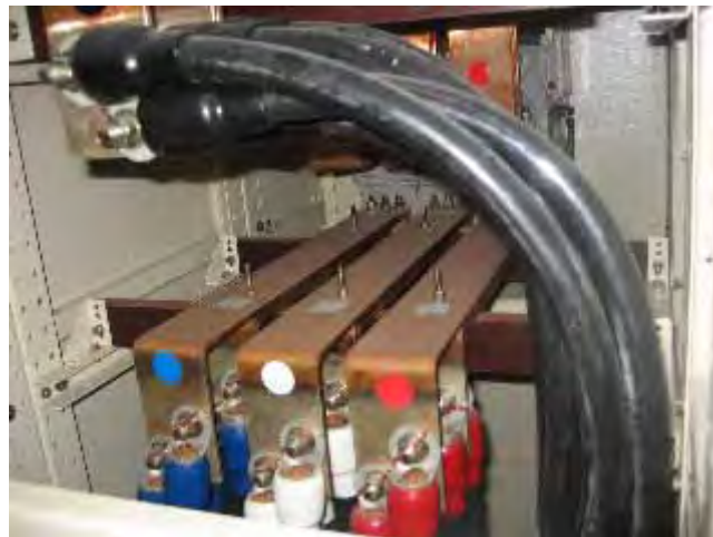
Fig. 2.2.2-5 Inside of the main distribution board in Palau International Airport
