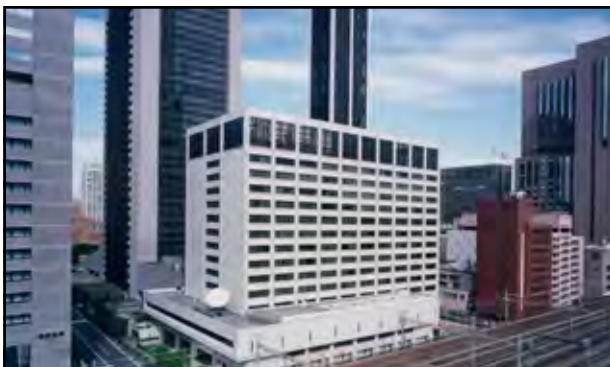
Tokyo Electric Power Company Head Office Building: The managerial function of TEPCO, and its central function of power supply are placed in the building.
