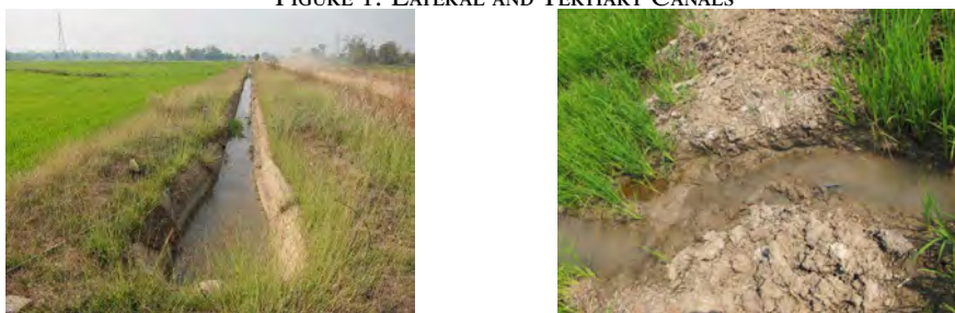
FIGURE 1: LATERAL AND TERTIARY CANALS
