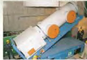
500kV GCB(Gas Circuit Breaker)Installation
