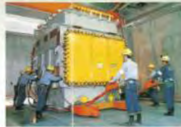
Transformer Installation
