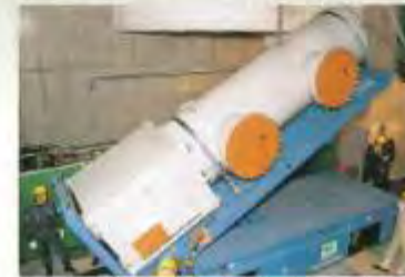
500kV GCB(Gas Circuit Breaker)Installation
