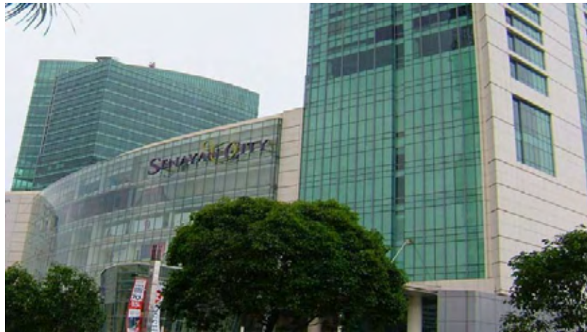
Figure 4.4-3 Photograph of a Commercial Building
