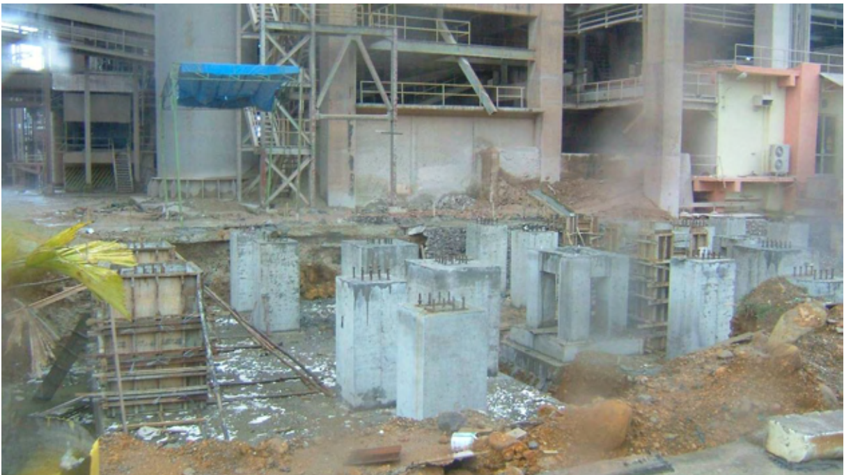
6) Site for Waste Heat Recovery boiler installation
