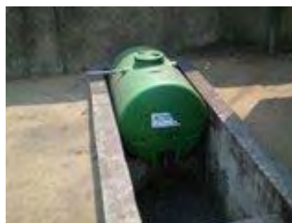
Empty water reservoir
