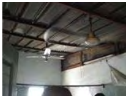
Roof of consultation room
