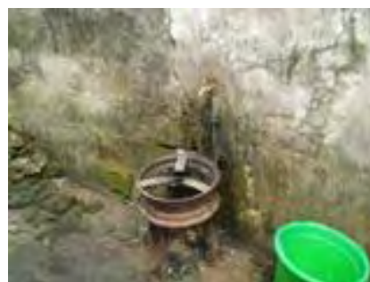
Water supply outdoor
