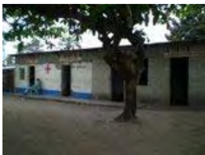
Exterior of health center
