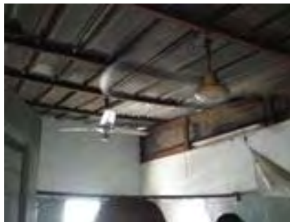
Roof of consultation room
