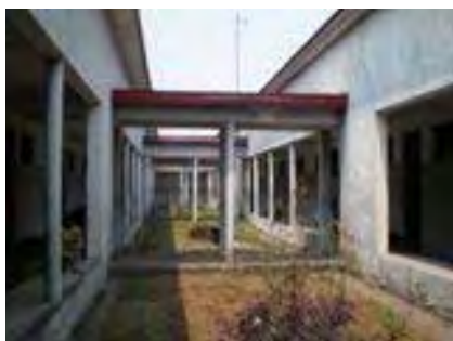
Maternity-ward and court-yard
