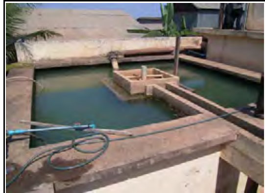
Photo 4-2 rapid coagulated sedimentation method is employed as treatment method but as this method needs high operation skill, treatment efficiency is poor.
