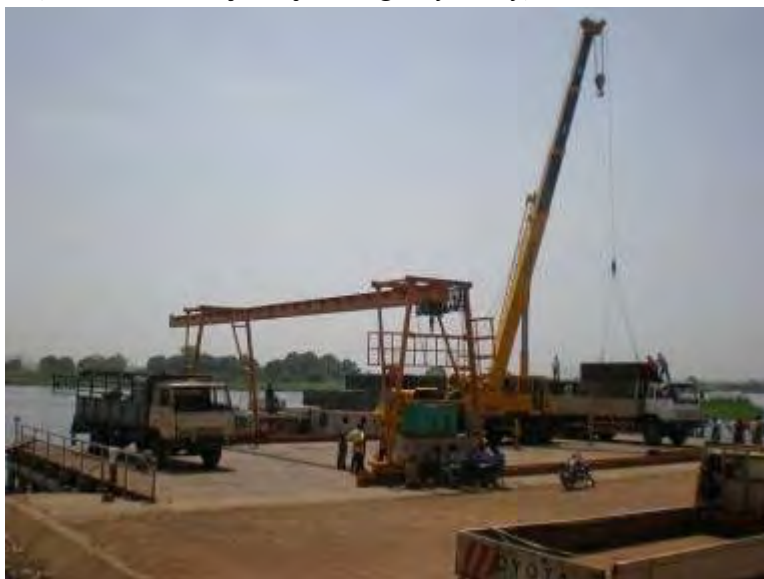
Jetty & Cargo Handling Yard
