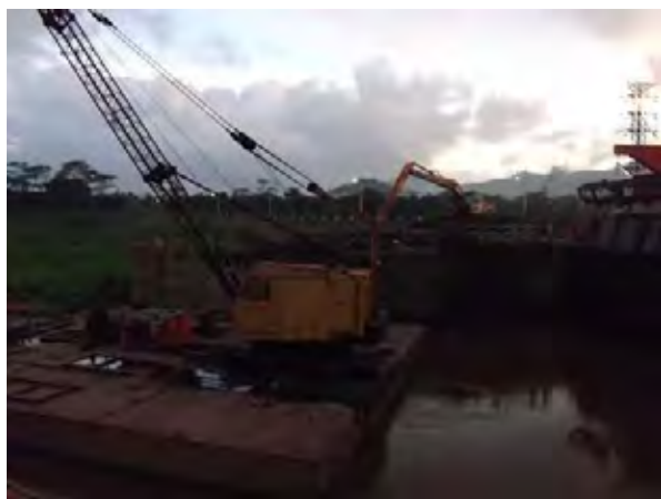
Sengguruh Dam - Garbage Removal
