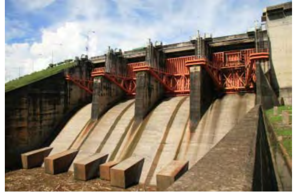
Spillway Gates
