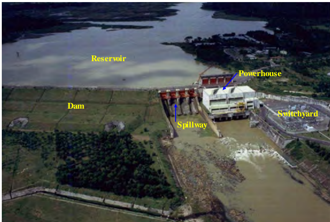
General Layout of Wlingi Power Station
