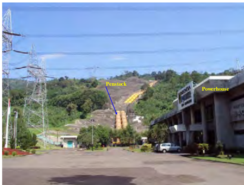
Saguling Power Station
