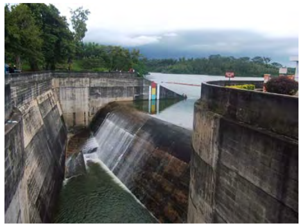
Lahor Dam - Side Spillway
