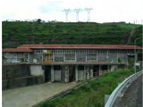
Soedirman Hydropower Station
