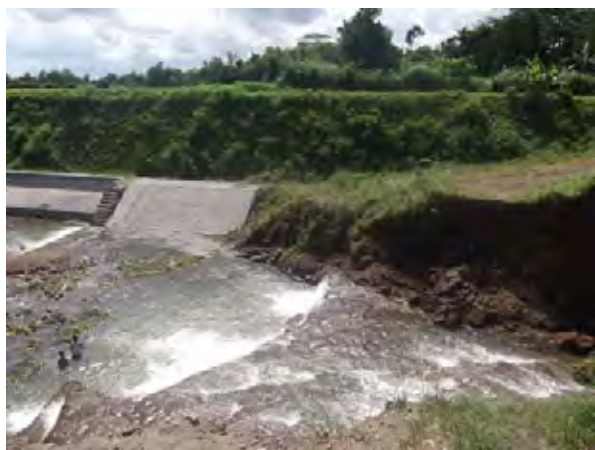
By-pass Channel Located Upstream of Wlingi Dam
