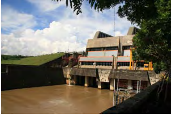
Wlingi Hydropower Station
