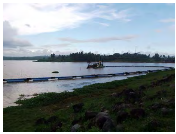
Reservoir - Dredging Works
