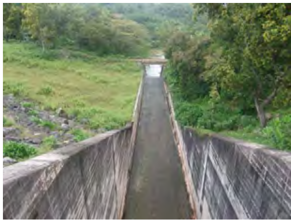
Lahor Dam Spillway - Chute Way
