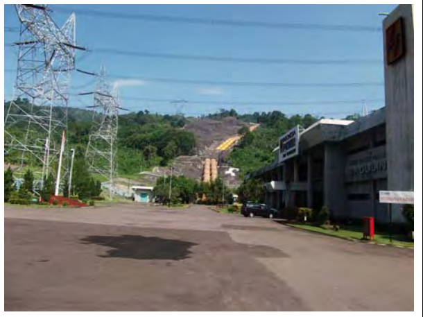
Power Station and Penstock Line
