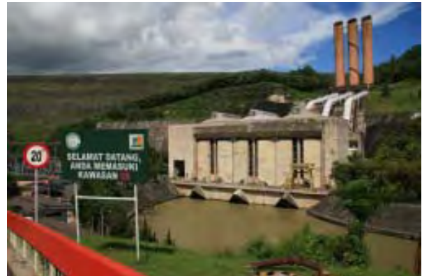
Sutami Hydropower Station
