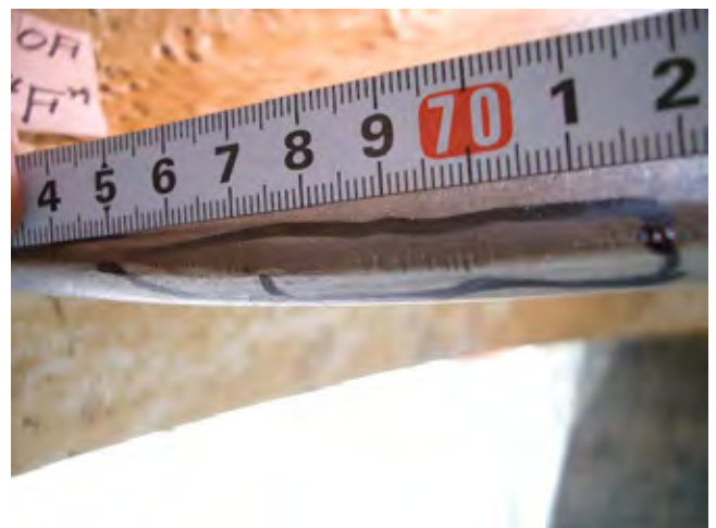
Cavitation at Outlet Side
