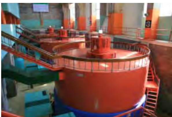
General View of Power House
