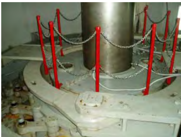
Water Turbine Pit
