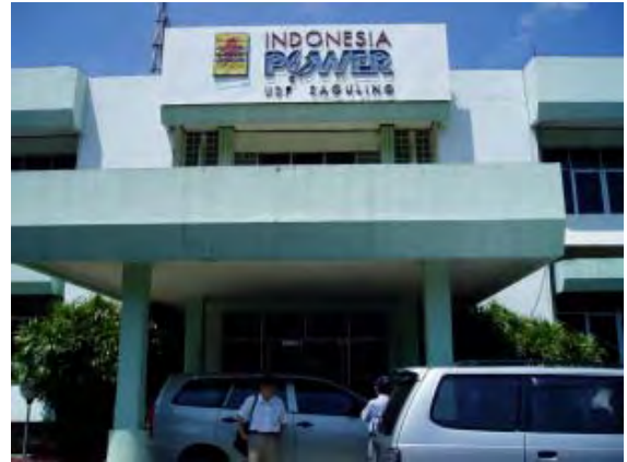
Saguling Hydropower Station
