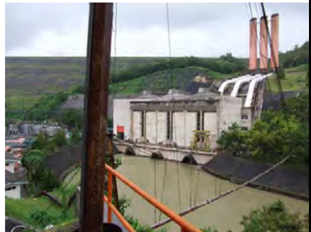
Power Station, - Tailrace Channel
