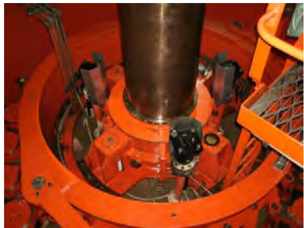
Water Turbine Pit
