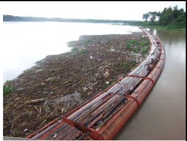
Reservoir - Floating Log Boom
