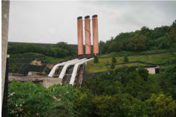
Sutami Hydropower Station
