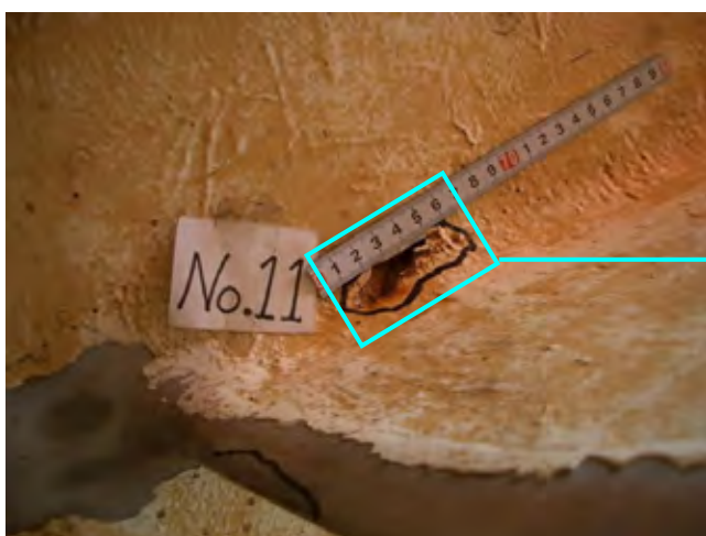
Pitting Corrosion at Outlet Side (Only on Blade No. 11)
