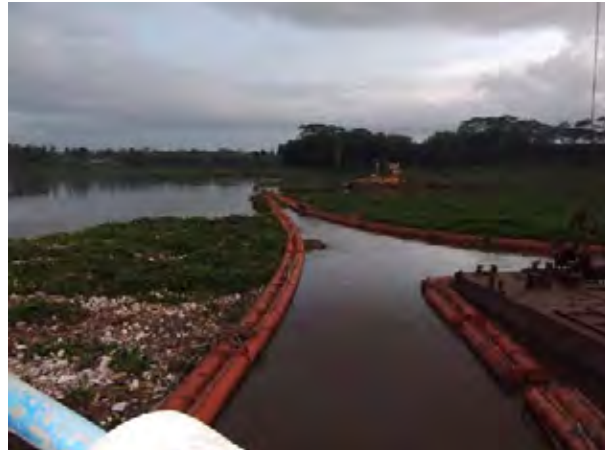
Sengguruh Dam Reservoir - Floating Log Boom
