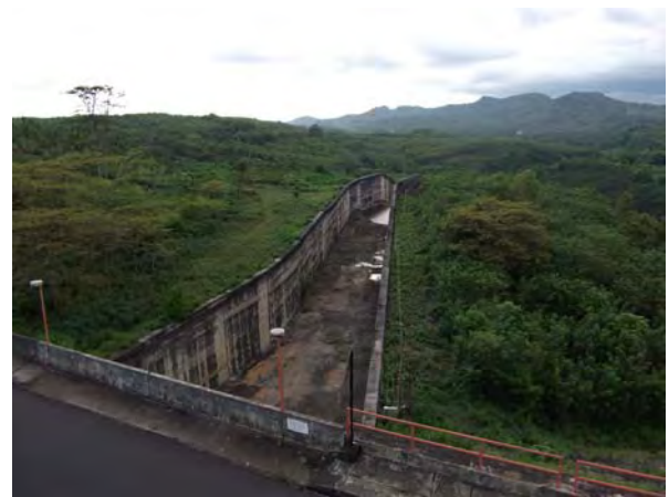
Spillway - Chute Way
