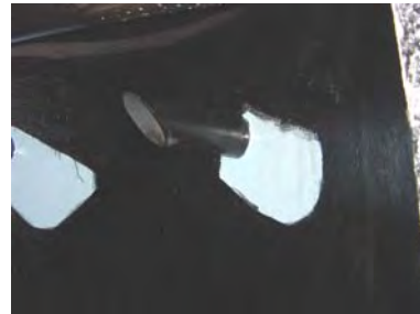
Aeration Pipe (Upper Draft Tube)
