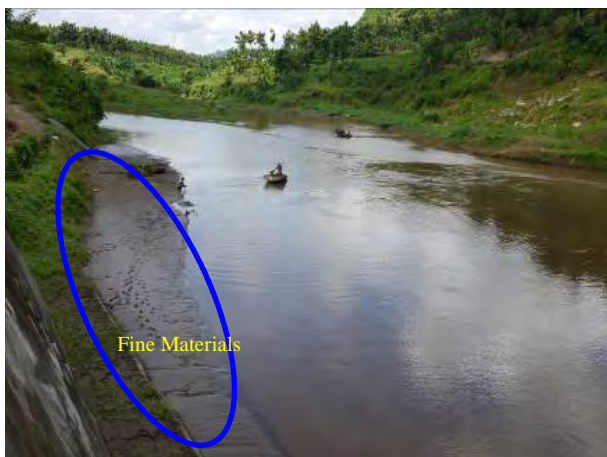
Just upstream of the newly constructed Sabo-dam in Lesti River. The reservoir is filled by fine materials, such as sand, silt, clay.
