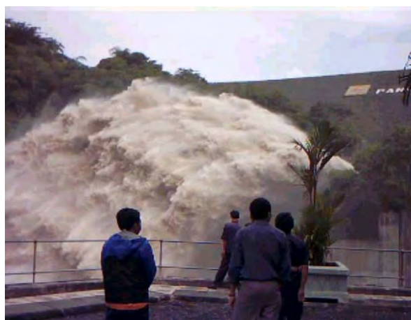
Sediment Flushing Operation from Mrica Dam (Prepared by Indonesia Power)
