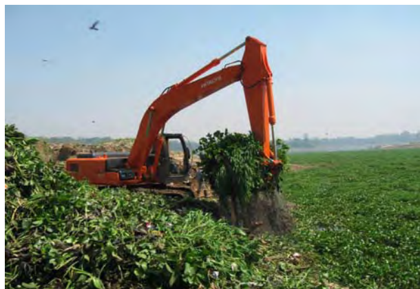
Disposal operation of water-hyacinth in Saguling reservoir
