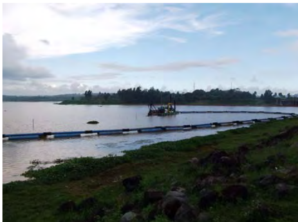
Wlingi reservoir, Reservoir dredging works
