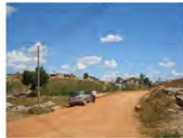
837 Power Cable Line
