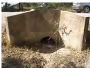
812 Pipe Culvert D600
