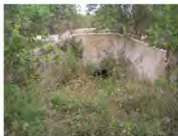
813 Pipe Culvert D600
