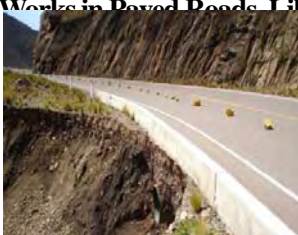
Collapse of drainage
