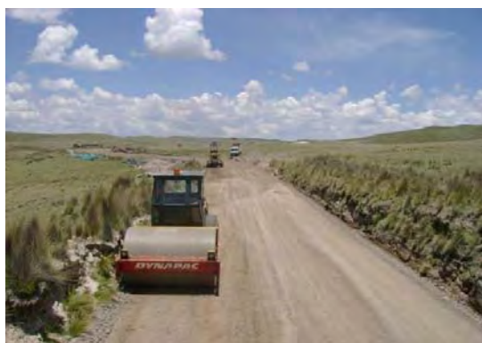
Sub-base Compacting
