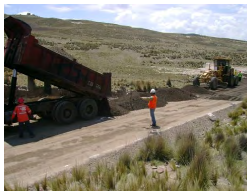
Settling and Extending Stabilized Base
