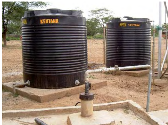
井戸とフッ素除去装置の Born Jar が 2 槽
