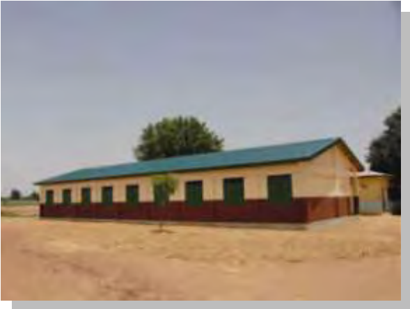
Completed New School Building Bagauda Primary School, Bebeji LGA
