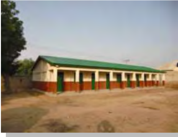
Completed New School Building Kawaji Jigiriya Primary School, Nassarawa LGA
