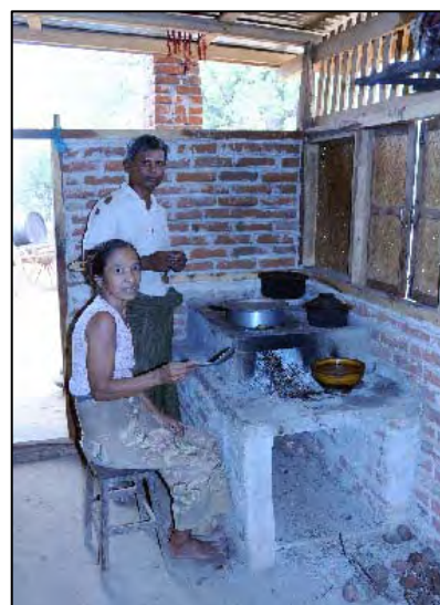
Photo 4: An elevated cooking stove constructed by a villager.
