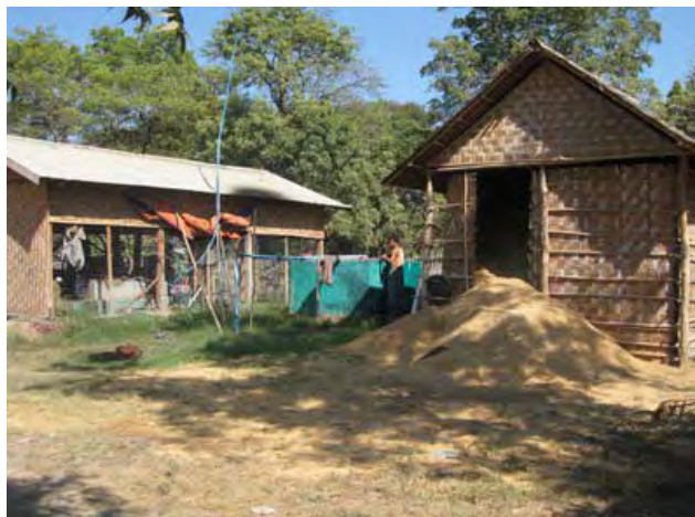
Photo(2) - A paddy-husk storage was built by under arrangement of the Committee beside the paddy-husk bio-gas' building
