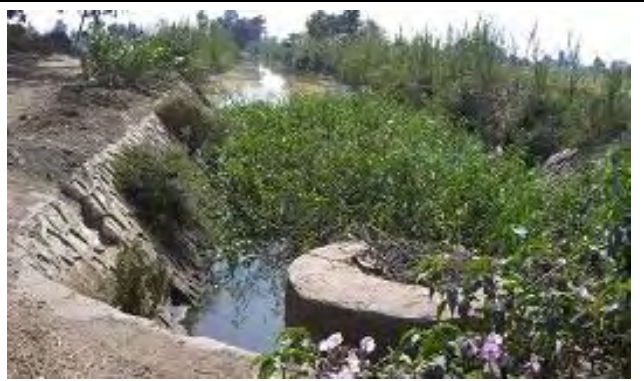
End point of Bahar El Nour irrigation canal
