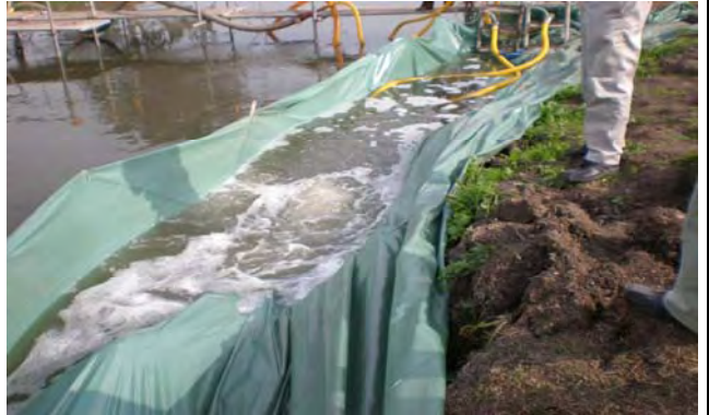
12. MBD operation in temporary drain
