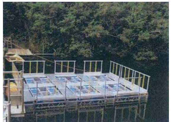
Float type aquatic plant treatment facility
