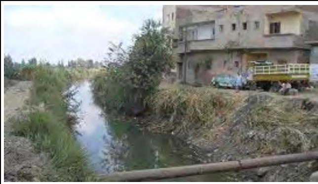
Bahar El Nour irrigation canal at Al Saei village
