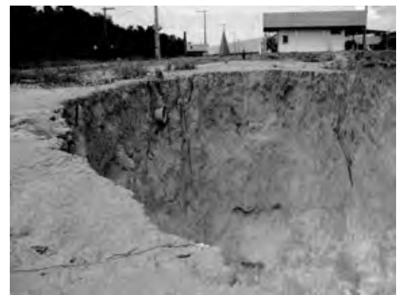
Erosion in the area is a major concern.
