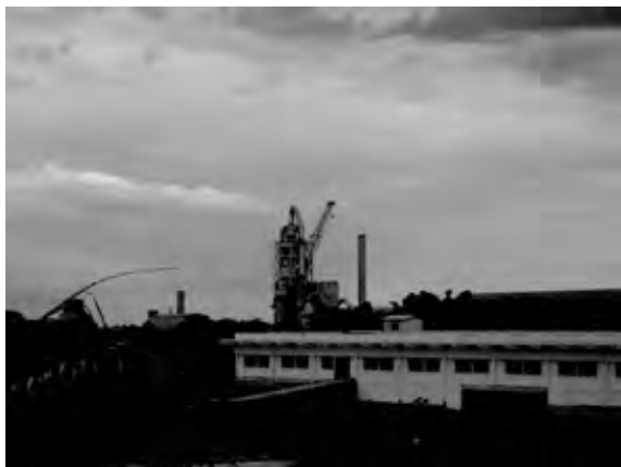
A cement factory in Manaus.
