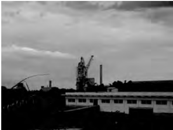
A cement factory in Manaus.
