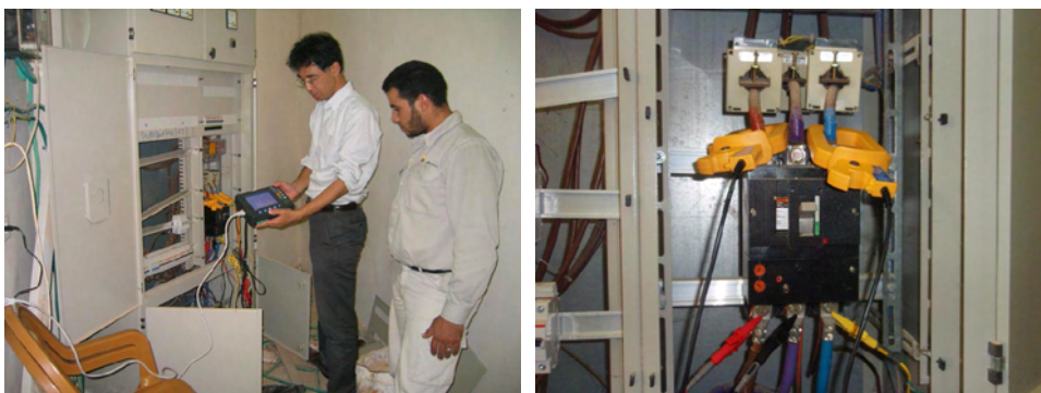
Photo Left : Measuring voltage and frequency
