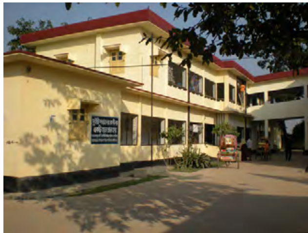
Shorail UHC, Bramanbaria
