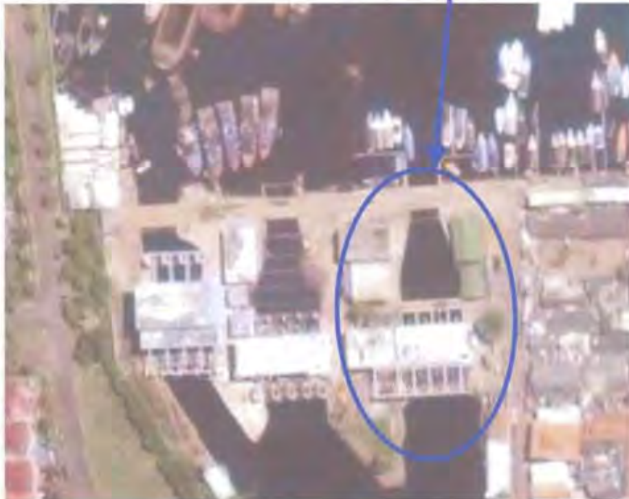
Pluit Pump Station
