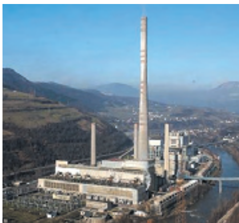
Kakanj Thermal Power Plant
