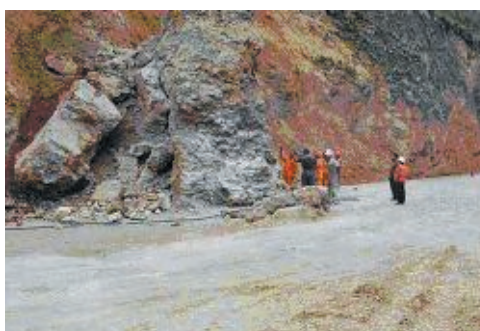
Rock Clearing works (Jauja-Tarma section, Junin Region)
