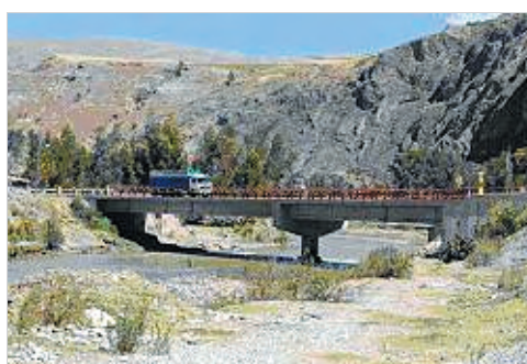
Bridge constructed under the project (Junin Region)
