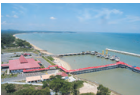
Ferry terminal constructed under this project (Muntok)
