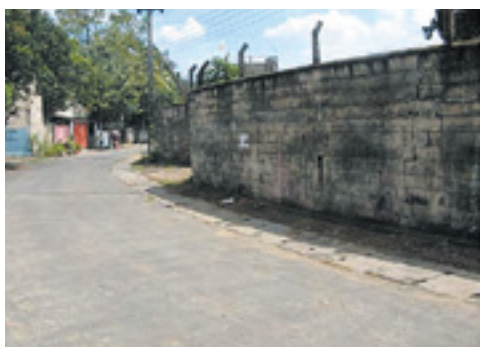
Side drains with slab lids requiring easy operation and maintenance (Attidiya)
