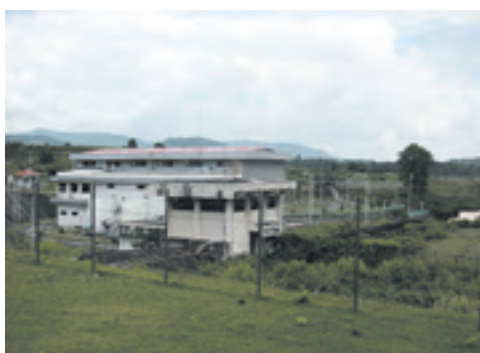
Bili-Bili Power Plant
