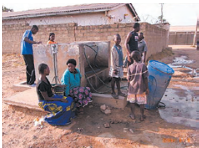
N'gombe unplanned settlement in Lusaka (residents collecting water from communal tap developed with Japanese Grant Aid)
