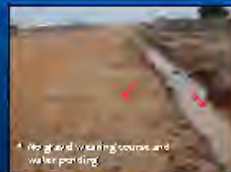
1. No gravel wearing course and drainage away and sidewalks 2. No gravel wearing course and drainage away and sidewalks
