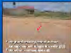
1. No gravel wearing course and drainage away and sidewalks 2. No gravel wearing course and drainage away and sidewalks
