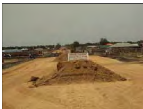
Barricade by earth and sign boards
