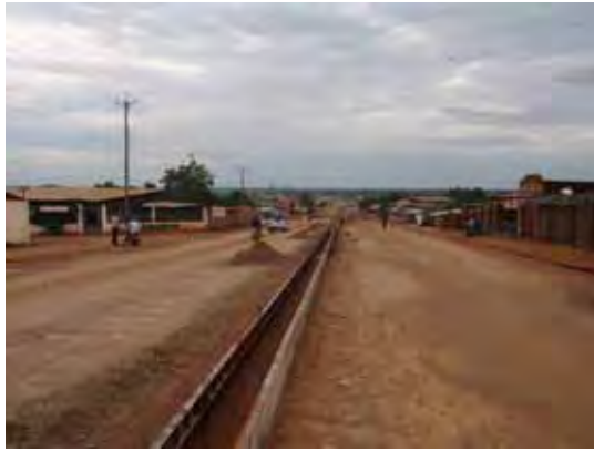
a. On-going Emergency Road Rehabilitation
