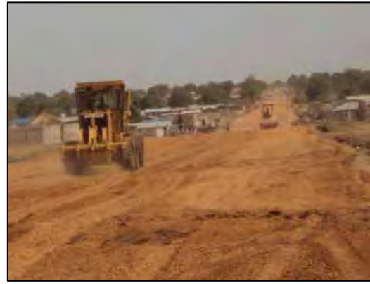
Spreading and Compacting
