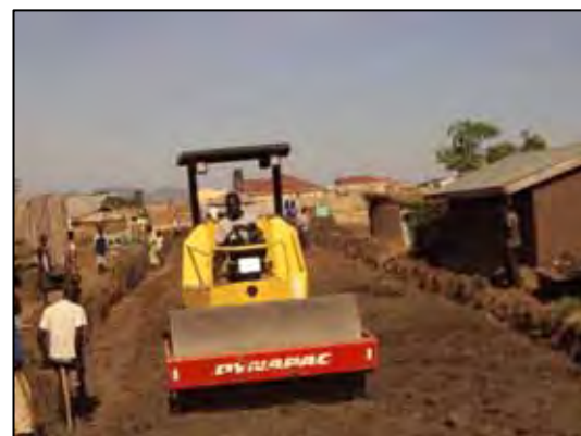
Construction of 10m Road
