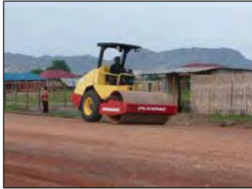
Compaction by a Roller
