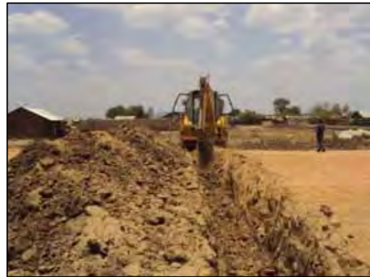
Trenching for Culvert
