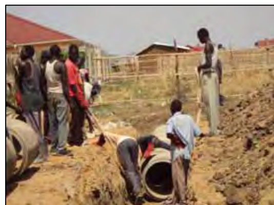
Setting of culvert
