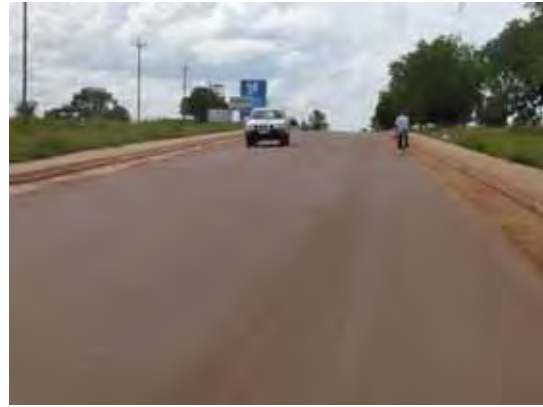
b. Asphalt Paved Road
