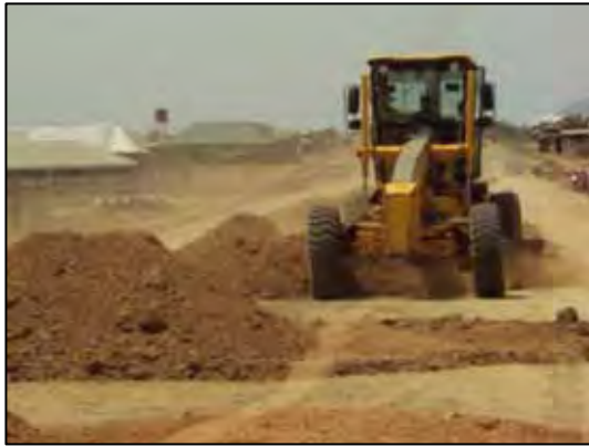
Spreading of Gravel
