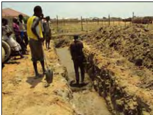
Making Culvert Base
