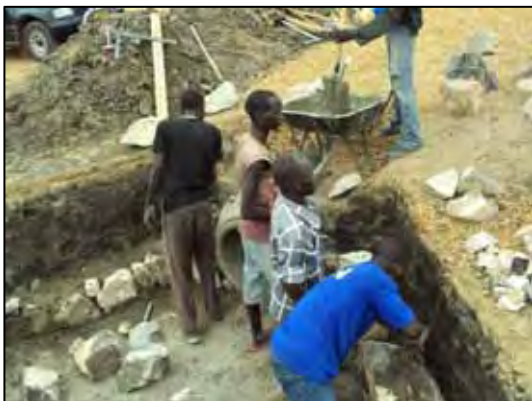
Making of Culvert Wing Wall
