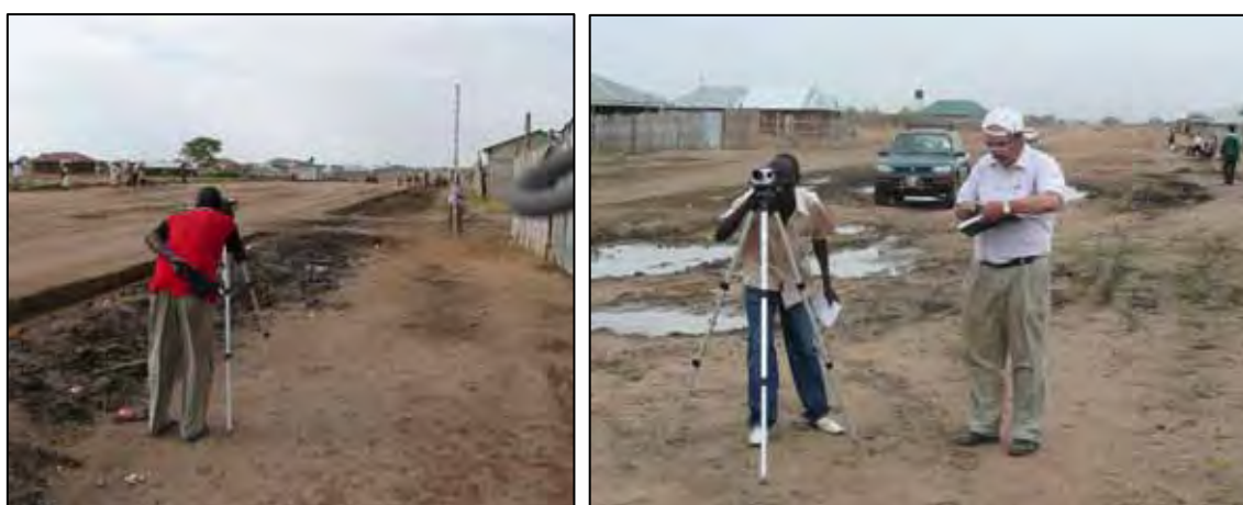
Photo 25.4.2-1 Survey Practice on Site
