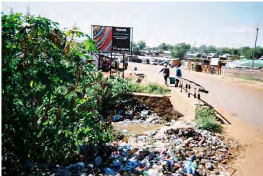
Photo 23.2-4 No.17 Bridge - Dumped and Accumulated Unsanitary Garbage
