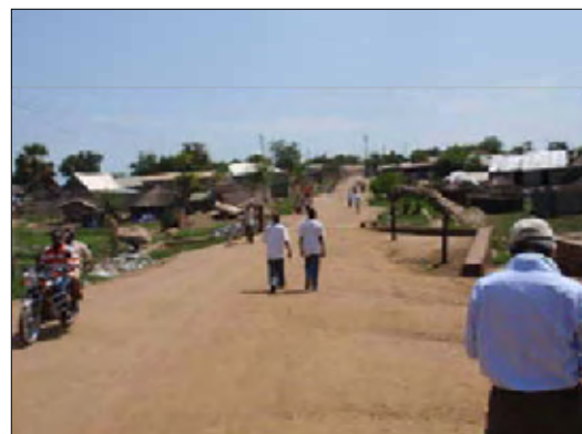
Narrow Bridge without Pedestrian Sidewalk (No. 4)
