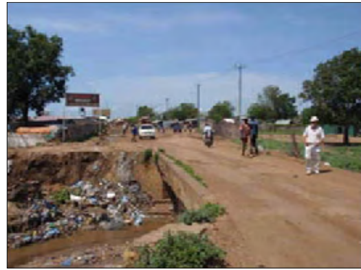
Narrow Bridge on Arterial Road without Pedestrian Sidewalk (No. 6)
