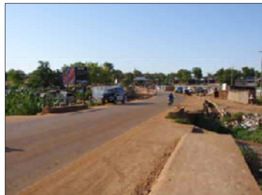
Road Narrows at Culvert Section of Paved Road (No. 17)
