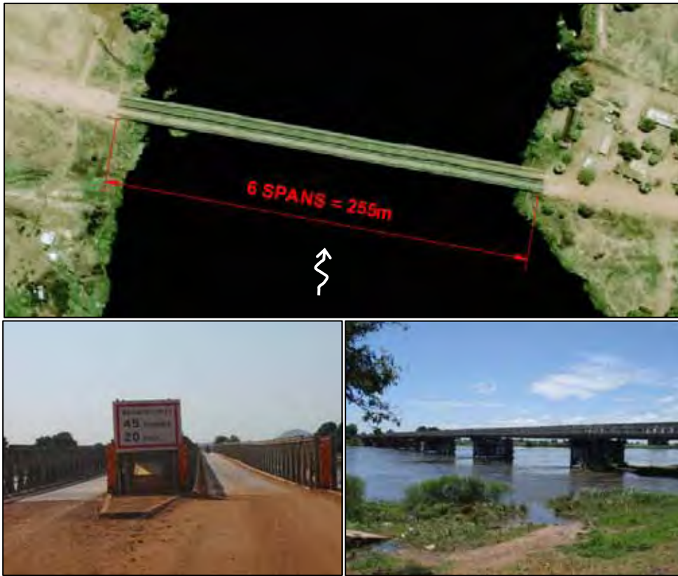
Figure 19.4.6-6 Existing Juba Bridge
