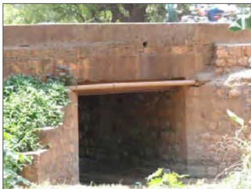
RC Slab on Steel H-Beam Culvert with Masonry Abutments (No.9)
