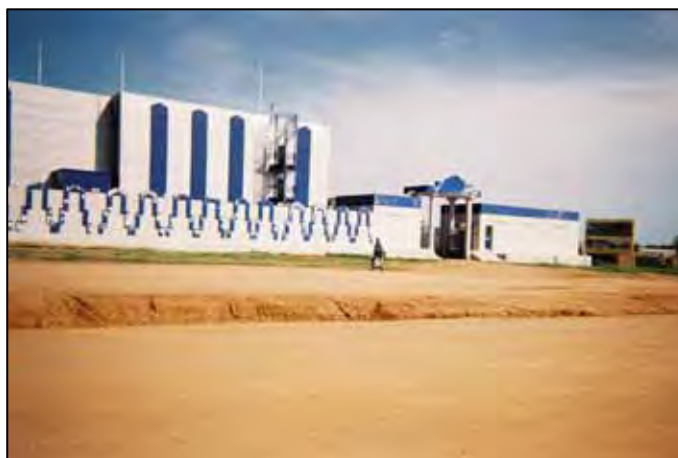
Photo19.6.2-6 New building of Ministry of Defense (in southern Nyakuron)
