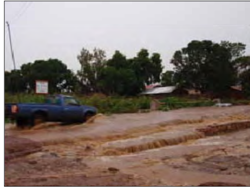
Floodwater Overtopping Bridge During Rain (No.12)
