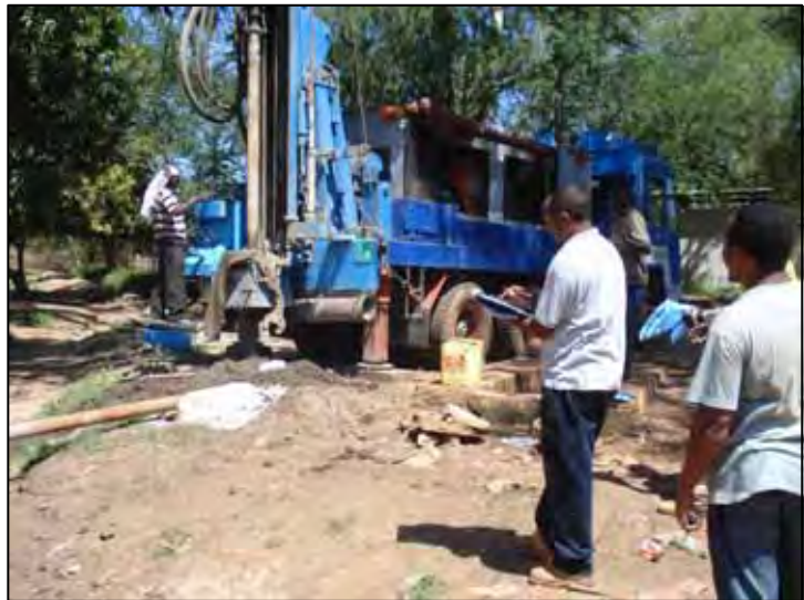
Photo 21.2-1 Drilling and Soil Profiling
