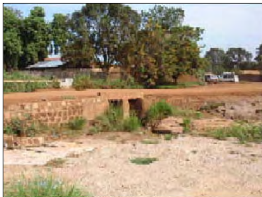
2-Cell RC Slab Culvert on Masonry Walls and Abutments (No.12)
