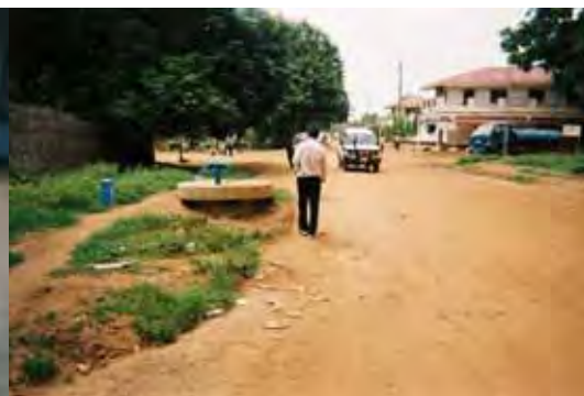
Photo 17.7.2-2 Water facility (Automatic Valve) along CR2-4
