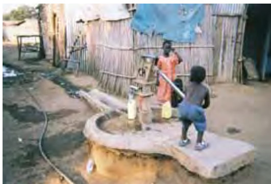
Photo 17.7.2-1 Well along CR9-2
