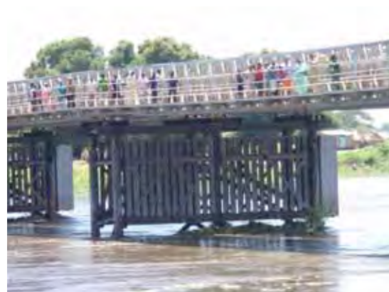
Steel Pile Bent Piers
