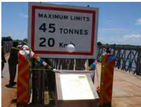
Load Limit Posted at 45 Tons (20 km/hr) During Juba Bridge Inauguration (Oct. 6, 2008)
