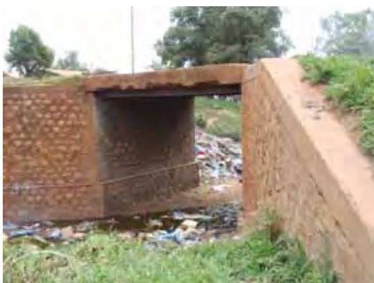
Typical 1-Span RC Deck on Steel H-Beam with Masonry Abutments
