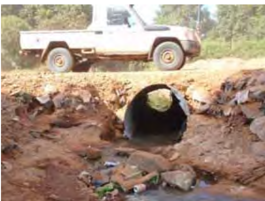
Typical Corrugated Steel Pipe Culvert
