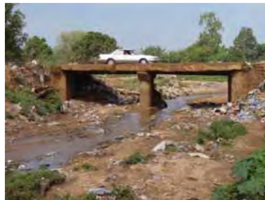
Typical 2-Span RC Deck on Steel H-Beam with Masonry Abutments and Pier
