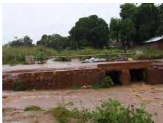
Typical 2-Cell RC Slab with Masonry Abutments
