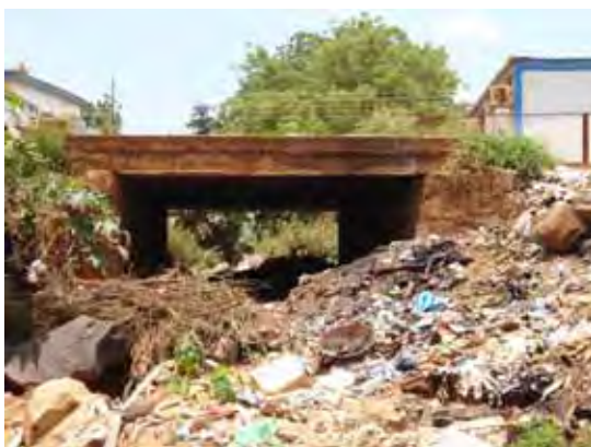
Typical 1-Cell RC Slab with Masonry Abutments
