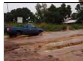
Bridge No.12 – Overflow during heavy rain
